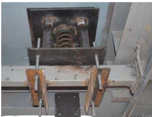
Fig. 10: Friction damper.
