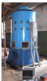
Fig. 1: Electric motor of a pump aggregate.
